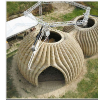
Sustainable 3D Printed Habitats WASP Debuts TECLA, a New Circular Model of Housing
